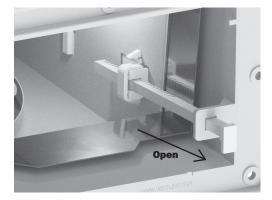
9. Reinstall damper, feeding the slide rod through the damper knockout opening. Verify damper operates.
